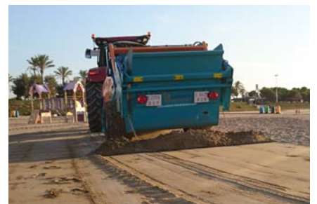
Final smoothing of the sand
